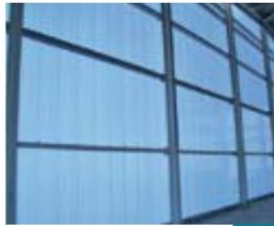
8 Wall Cladding Warehouse Lexan Thermoclick sheet system
