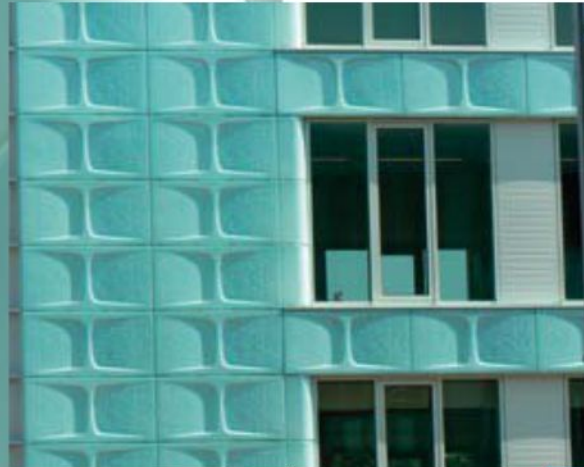
11 Philips Science Park Wall Cladding Lexan® SG305 SLG sheet
