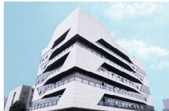
▲ Changsha Guangxiu Hospital, Hunan China
